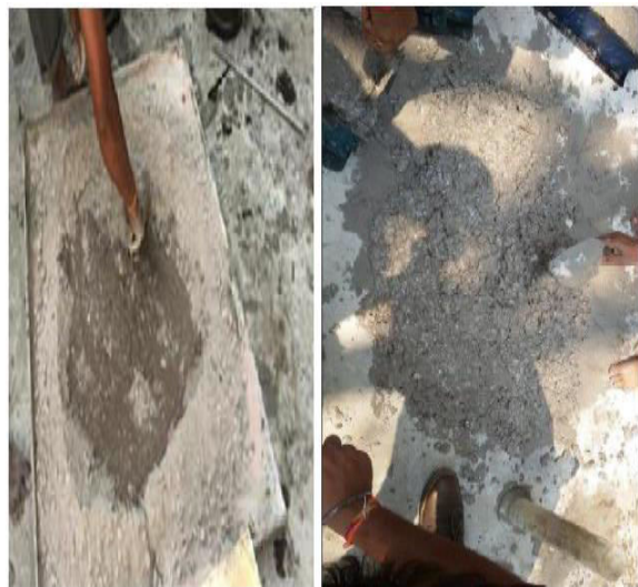
Mixing of Geopolymer concrete
